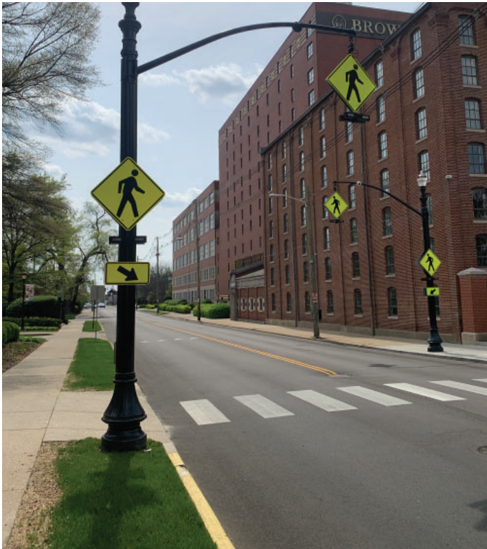
Well-defined pedestrian crosswalk and curb ramps along a main transit corridor. Location: Brown-Forman, 18th Street, Louisville, KY
