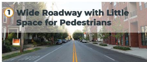
1 Wide Roadway with Little Space for Pedestrians This 40' wide intersection can be uncomfortable to cross and leaves very little space for pedestrians to walk alongside the roadway.
