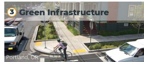
Through improvements to the streetscape, improvements to the stormwater infrastructure can also be developed. These vegetative beds can provide both functional and aesthetic benefits to the street.
