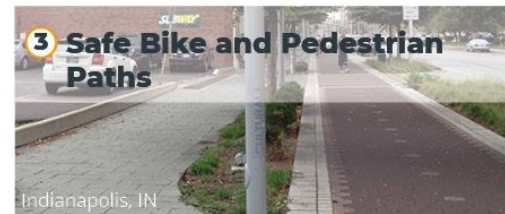
3 Safe Bike and Pedestrian Paths Indianapolis, IN Increasing the size of the sidewalk and adding a separate bike lane will eliminate conflict within the street and provide a safe space for pedestrians and cyclist to travel.
