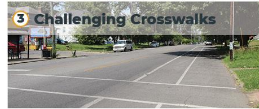
3 Challenging Crosswalks The crosswalks along this segment are typically 50' across making it difficult for users to cross in time and safely, especially when vehicles are traveling quickly.
