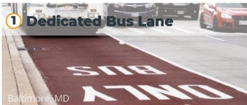
1 Dedicated Bus Lane Baltimore, MD By designating a lane of traffic to a bus route, you can eliminate the confusion of how bus, bike, vehicular, and pedestrian traffic interact with each other.
