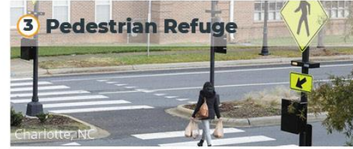
3 Pedestrian Refuge Charlotte, NC By implementing a pedestrian refuge in the center of the travel lanes, we can minimize the crossing distance while providing a safe pedestrian experience.
