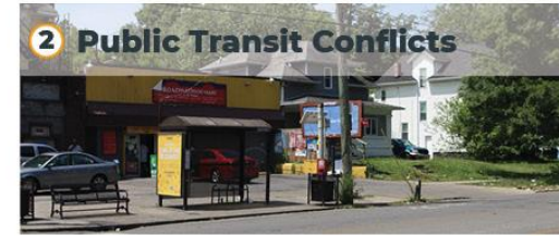
2 Public Transit Conflicts Public transit is available, but has inadequate space for stops. These areas also lack shade and proper lighting.
